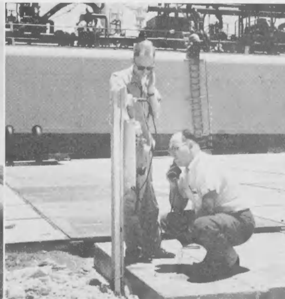
THE TWO men who connected the lines to the ammonia carrier were Calvin Schmidt and Adriaan Wever. Pumping ammonia aboard the Esso Centro America actually began at about 5:30 p.m., Aug. 3. Moments after the pumping had been started, the pipes, above, turned white with frost caused by the extremely low temperatures which keep ammonia in a liquid state. In sixteen hours, 4000 tons of Aruba ammonia were loaded aboard the carrier.
